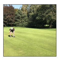
2) The centre line is marked with micro borehole locations 1m apart. Additional drill spots are positioned 0.5m between and perpendicular to the centre line to create a diamond formation.
