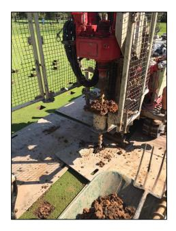
5) The groundwater recharge pumps are capped and inserted into the boreholes, the 1.5m and 3m drills are fitted with a single device and the 6m and 12m holes are fitted with an interlinked set of 3 devices. The devices have a 5-chamber tubular design made from polyethylene. Approximately 1,213metres of EGRP will be installed on the 8<sup>th</sup> green alone.
