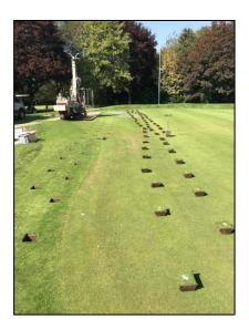
4) The centre line is drilled at either 6m or 12m depths and the offset drill spots are drilled to 1.5m or 3m. The micro-boreholes required to install the devices are 64-90mm in diameter. The greens surface is protected during drilling by using track mats. Any spoil is removed from the area.
