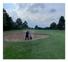
Once the bunker is shaped the base is compacted before the liner is installed.
