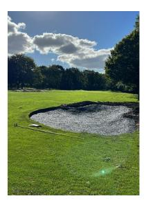
In this photo you can see a newly laid bunker liner, this is a mixture of crushed rubber and resin to for a liner that water get through but stop stones and soils from contaminating the fresh sand. Please stay out as much as possible, once laid it will take 24 hours to cure.
