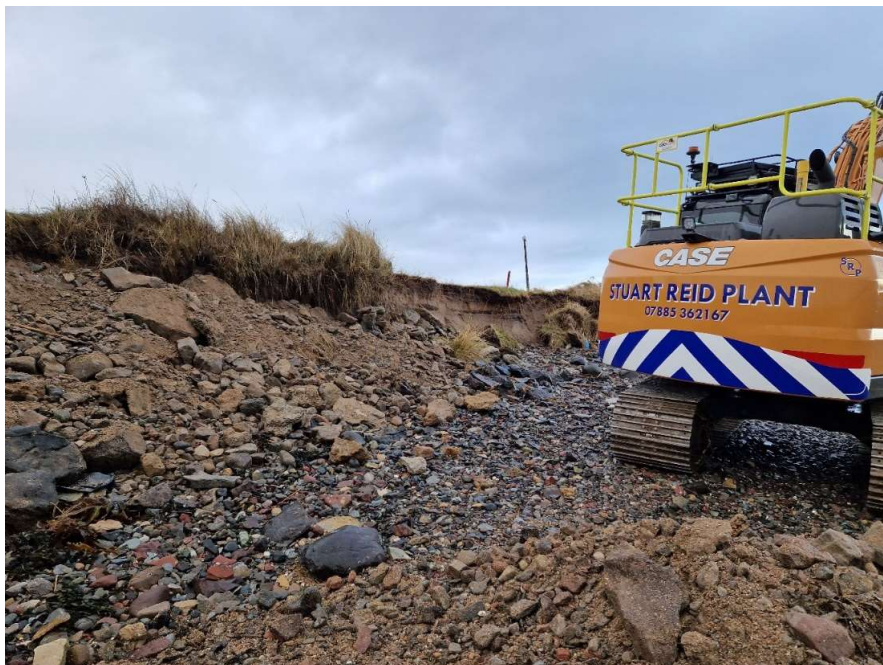
Figure 3: Stuart Reed building up the bank at the 3 rd tee.
