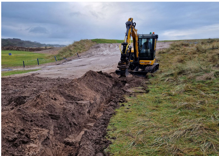
Figure 1: Richard Thorburn digging the irrigation trench on the 10 th path.
