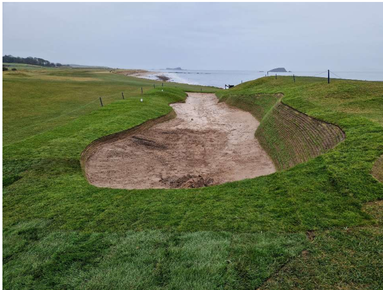
Figure 2: Turfing finished on the 17th.
