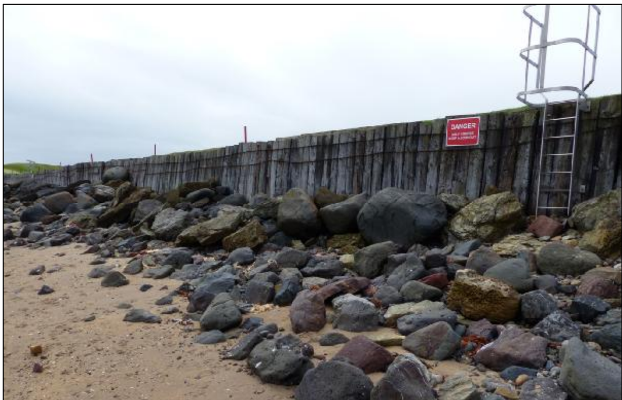
Vertical sleepered face and weak rock armouring protecting the 2 nd tees and carry area
