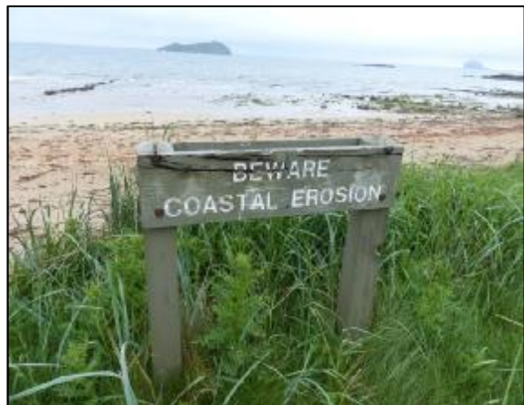
Coastal erosion sign 1 m from coastal edge
