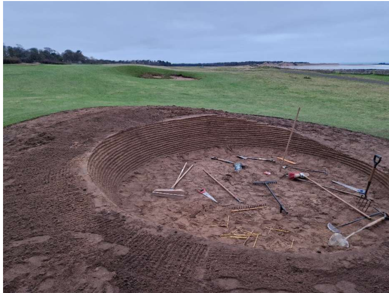
Figure 3: Rebuilding the front right bunker on the 5 th fairway.
