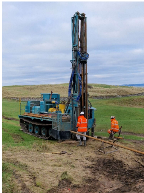
Figure 1: Drilling on the area outside of the greenkeeper's sheds.
