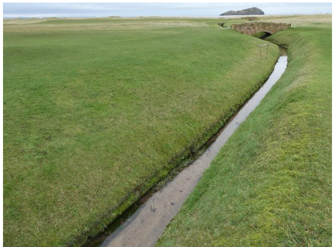
Burn with sleepered sides – note very shallow nature of the burn even though the water levels are relatively high
