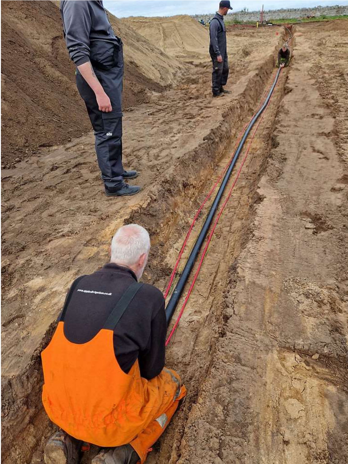
Pipe and cable being laid out
