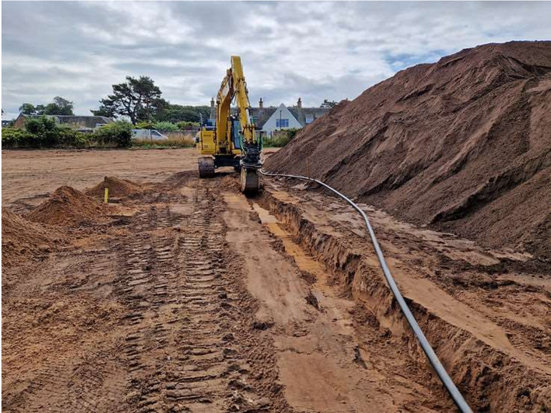
Alex digging the irrigation trench.
