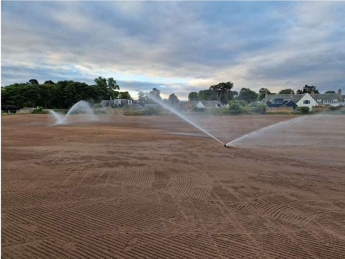
The irrigation system in action.
