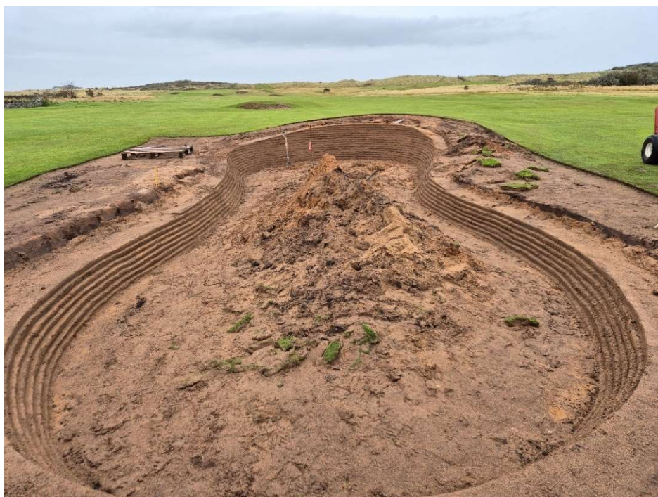
Figure 4: The revetted wall almost complete.
