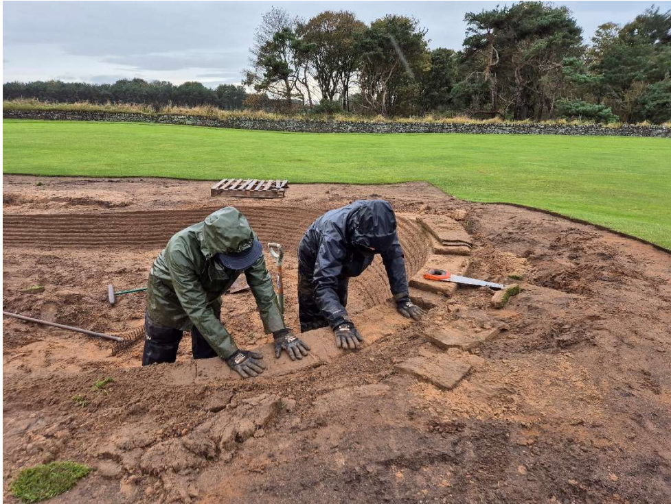
Figure 5: Graeme and Ryan placing in the top row after chamfering the edges.
