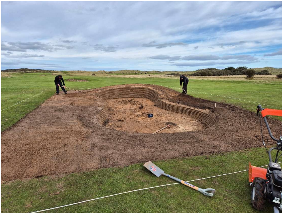
Figure 6: The 2 Ryans doing the landscaping works round the sides.
