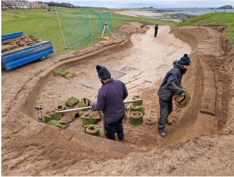
Figure 4: Luis and Rick laying a line of revetted turf.
