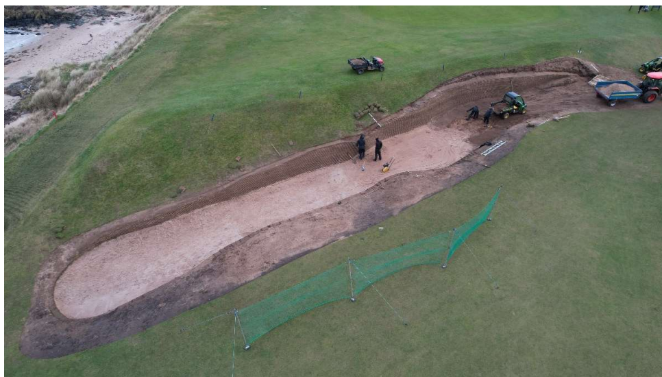
Figure 3: Sand being installed in the bunker.
