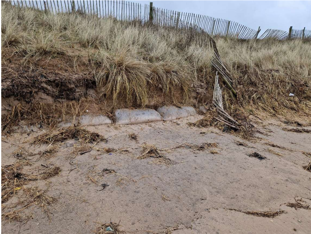
Figure 1: The exposed sandbags at the 11 th Coastal Protection area.
