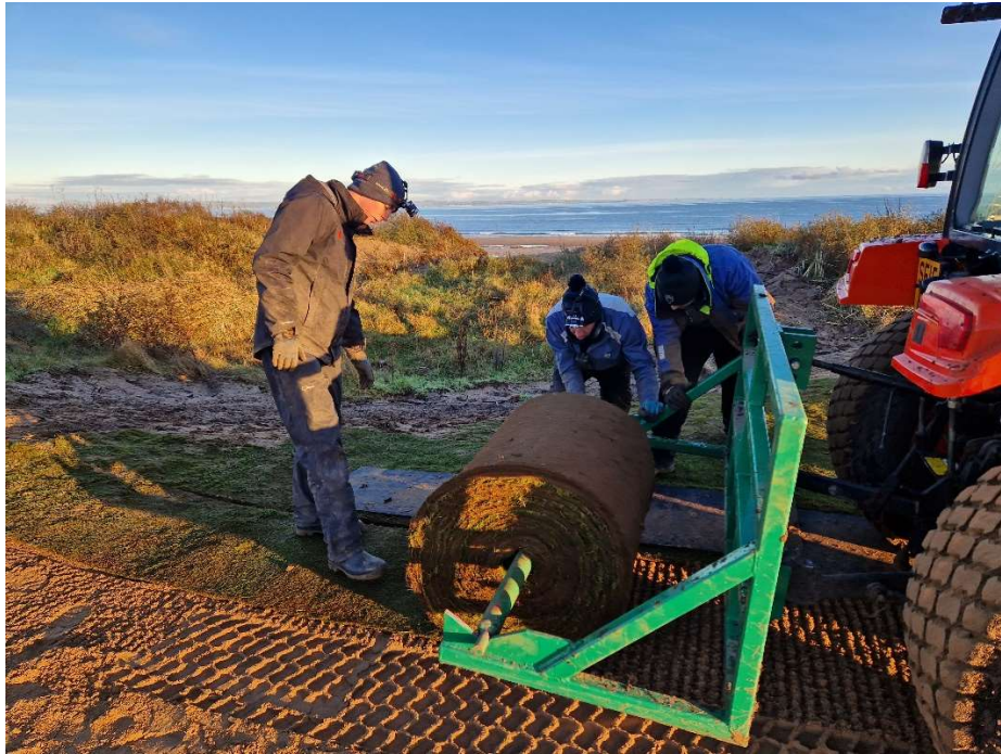
Figure 3: Big rolls being laid on 10 th tees.
