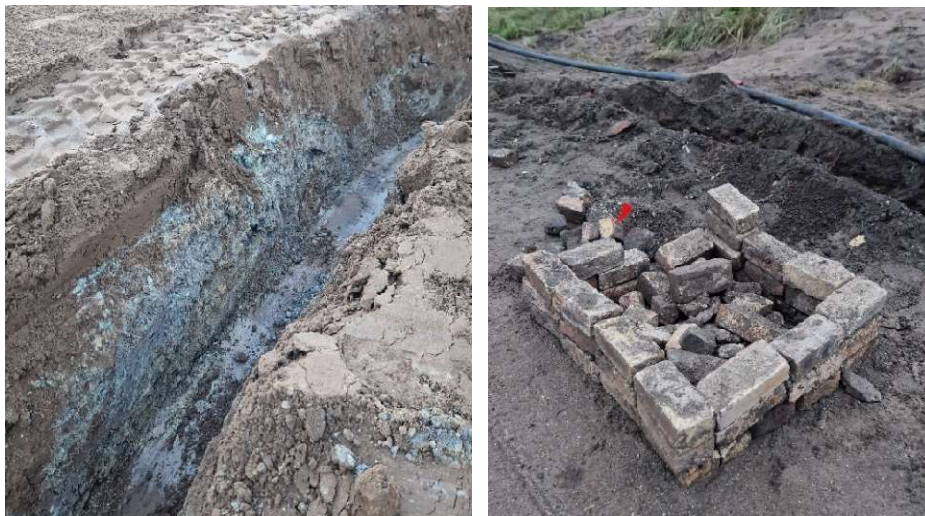
Figure 2: Poor subsoil on the 10 th tee with a pile of bricks pulled out by the trencher.
