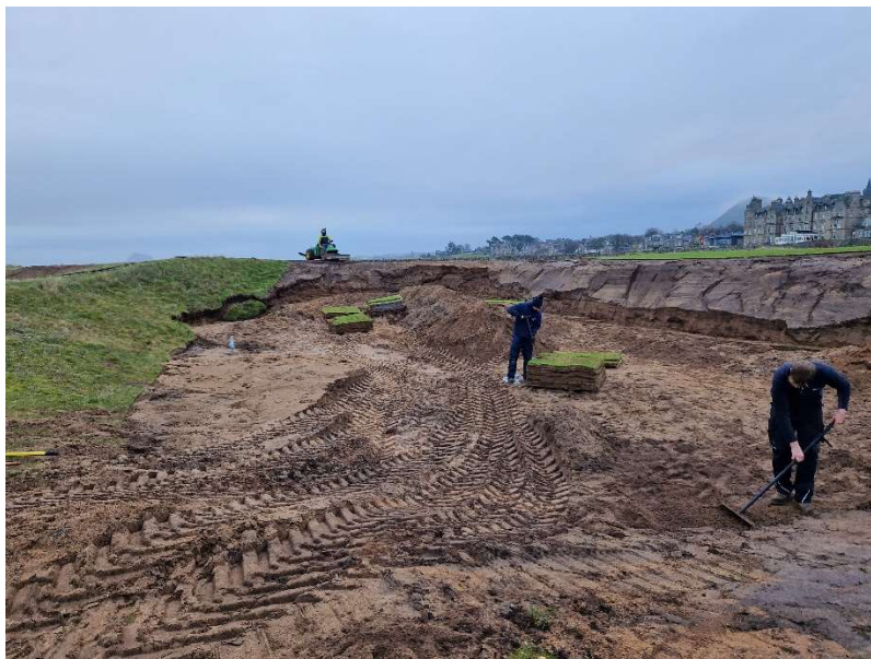
Figure 6: Renovated bunker on Redan.
