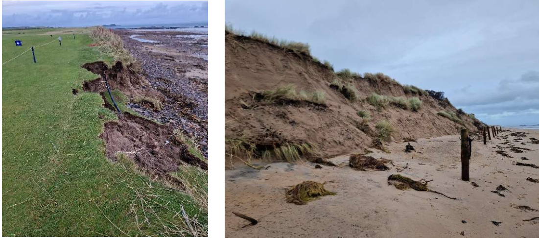
Figure 1: Coastal damage at 3 rd tee and dune on 11.
