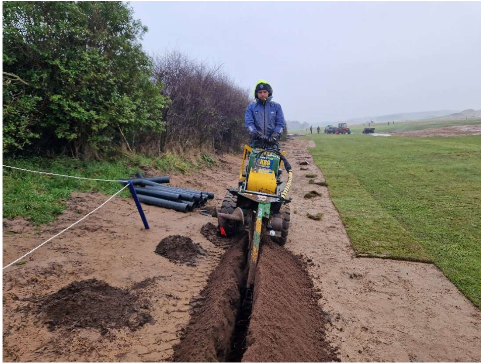
Figure 5: Graeme trenching the Irrigation line on 6 th tees.
