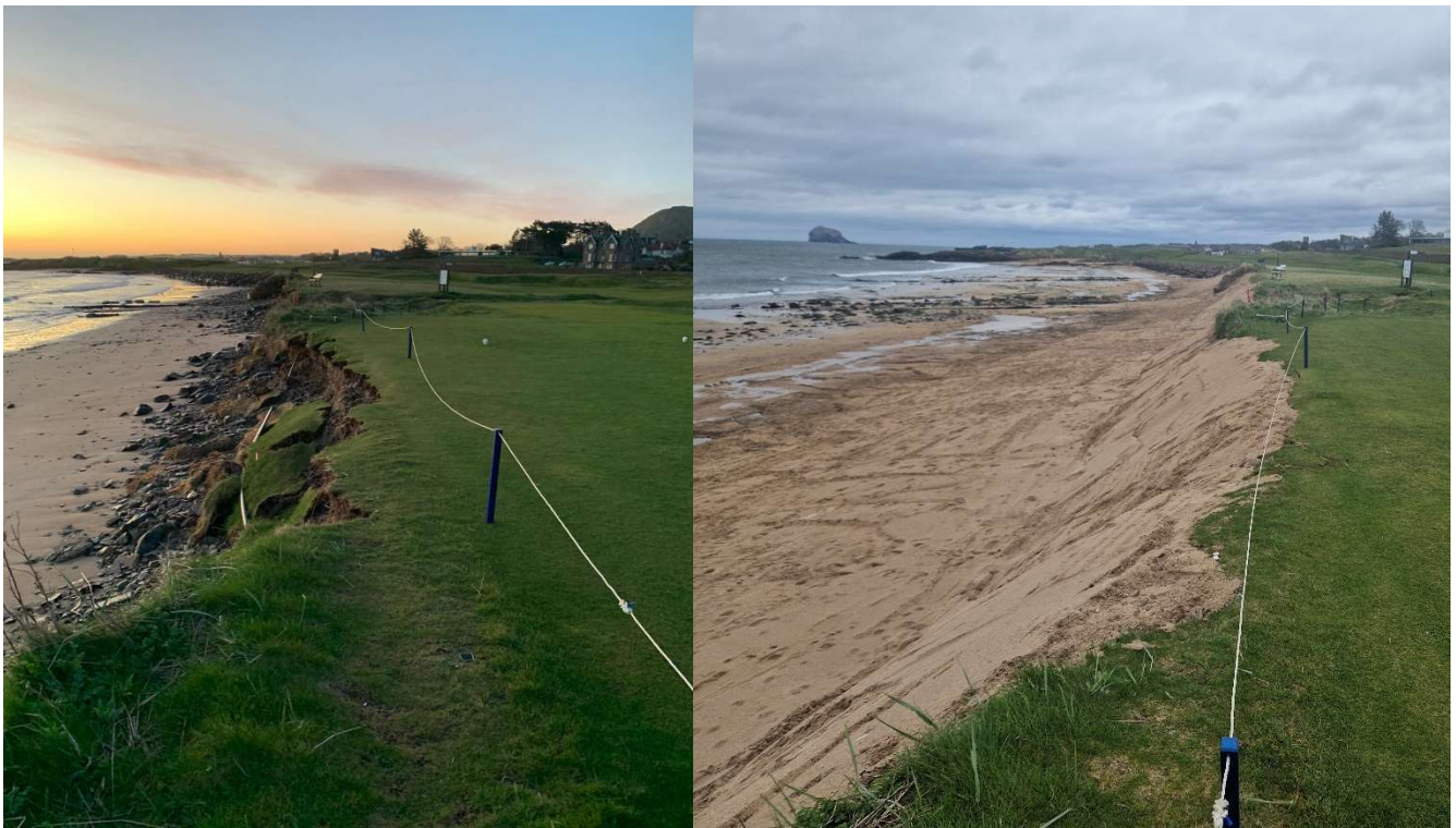
Figure 4: Remedial coastal erosion work at the 3 rd tees
