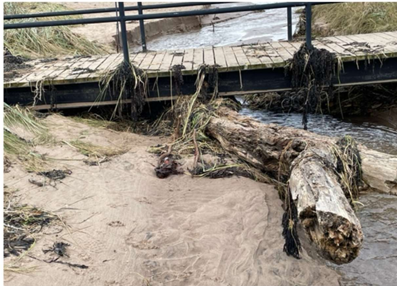
Figure 1: Tree trunk obstructing the flow of the Eel Burn
