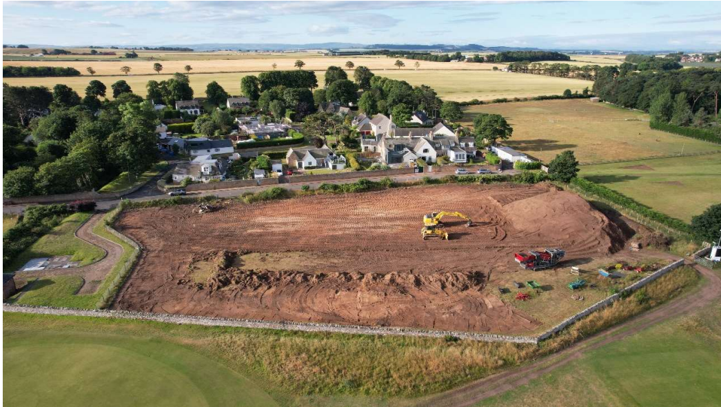
Figure 5: A few days into the clearance works – a stark difference already.
