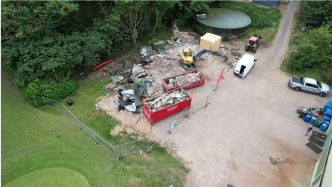
Figure 7: The Bulk Material Building during site clearance.
