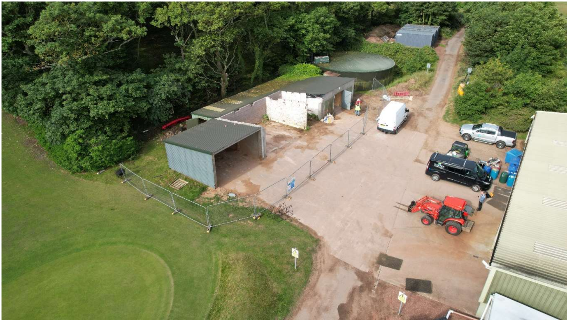
Figure 6: The Bulk Material Building before demolition.
