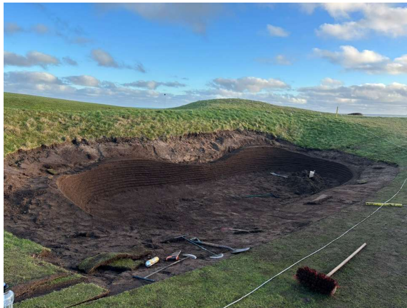
Figure 2: The right-side cross bunker on 14 with the revetted wall built.
