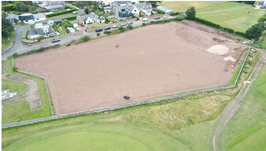
Figure 3: Turf Nursery being seeded by Greotech
