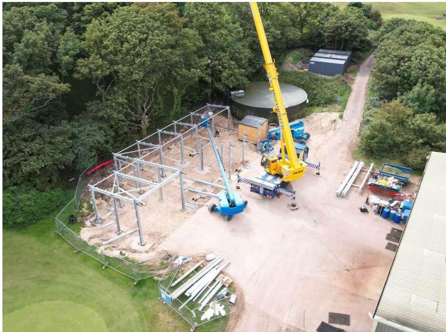
Figure 2: Steel framework being installed.
