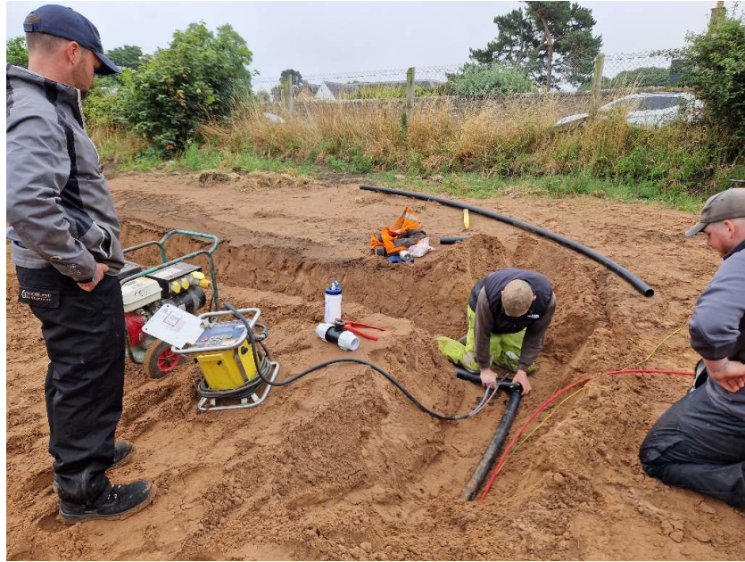
Figure 5: Graeme and Alex learning how to fusion-weld pipes together
