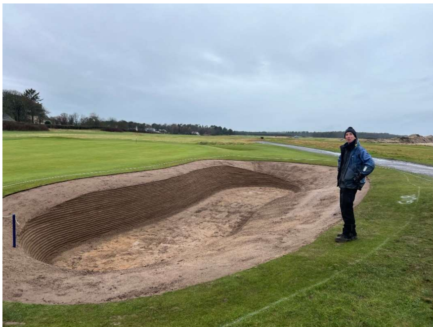
Figure 2: The bunker front right of 6 before being rebuilt. The walk-in on the left side of the photo was badly eroded and the face had been built inside the previous revetted wall.
