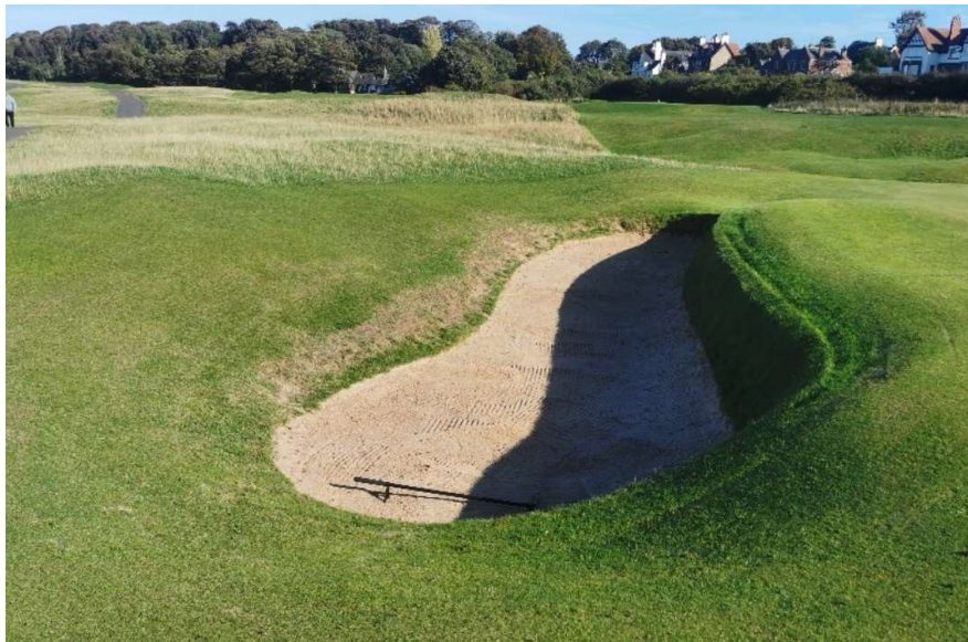
Figure 2: The bunker front right of 6 before being rebuilt. The walk-in on the left side of the photo was badly eroded and the face had been built inside the previous revetted wall.
