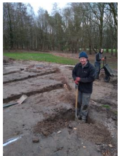
Hand digging the drainage channels at the 1st hole.
