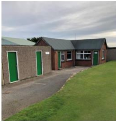
New doors on greensheds
