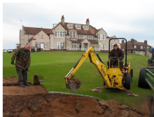
Work ongoing at 18 th bunker
