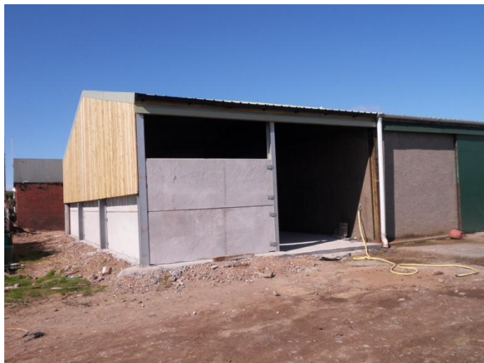
Soil Store extension almost complete.
